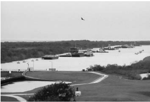
View of the traffic backup from the Colorado Locks Photos courtesy of Simon DeSoto
