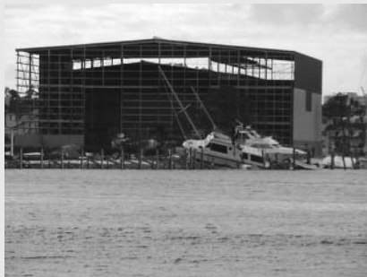
Extensive damage was visible from the Kirby responder's launch site
